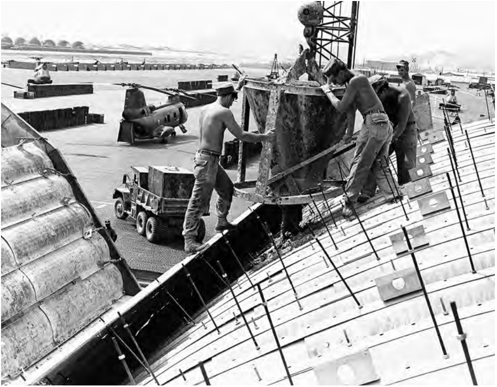
Seabees pouring concrete for Wonder Arches at Da Nang Air Base
